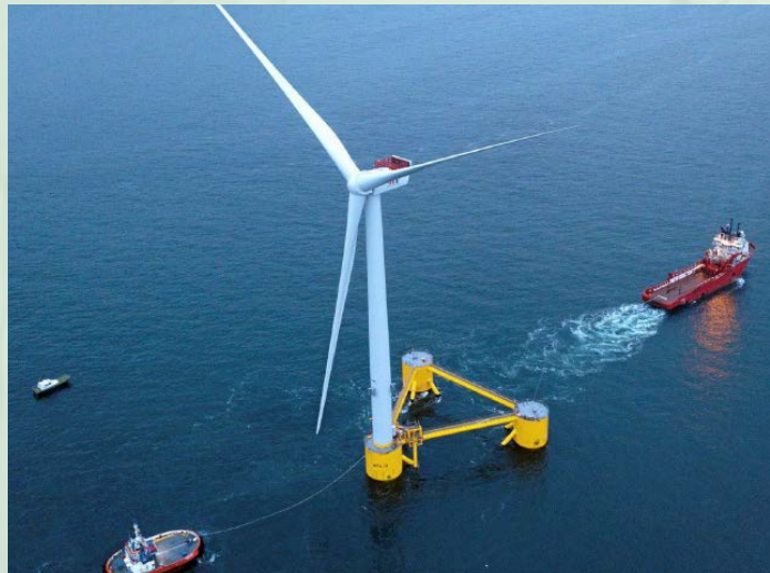
Off-shore wind turbines planned as a huge development in the South West
